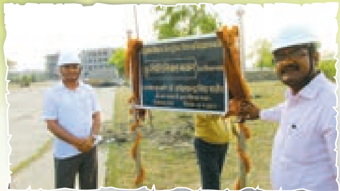
Foundation Laying of Vice-Chancellor's Residence
