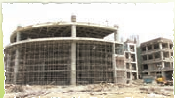
Earth, Biological & Environmental Sciences Building
